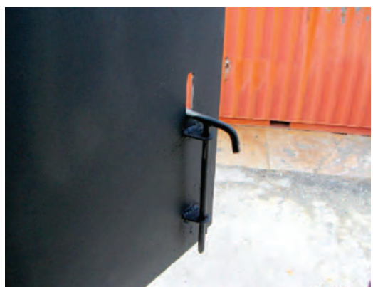
Figure C-6: Window & Latch Construction
