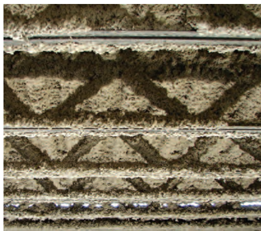
Figure C-4: Fireproofing added to structural steel
