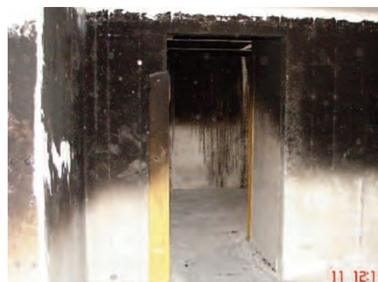
Figure C-7: Interior View of Burn Prop
